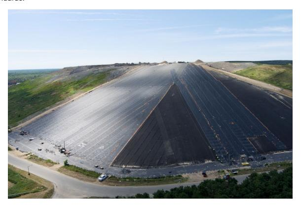
The project utilized **ClosureTurf® Advanced Revetment Technology**, a final closure system designed to provide long-term protection, efficient drainage, and enhanced environmental compliance.
