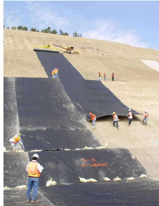
Challenging steep slope liner deployment
