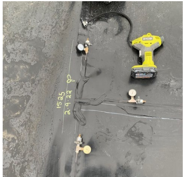
Figure 2 – Extrusion Fillet T-Seam - LLDPE
