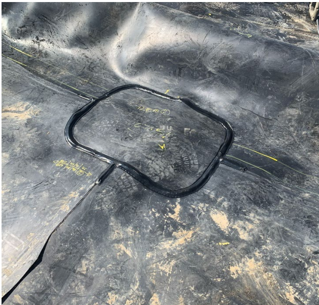
Figure 1 – Patched / Cap Strip T-Seam - HDPE
