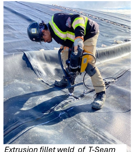
Extrusion fillet weld of T-Seam
