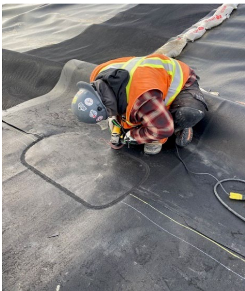
Photos showing grinding and extrusion welding of HDPE T-Seam patches
