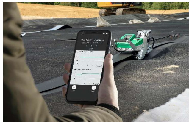
Leister GEOSTAR Data Control Welder with user App.
