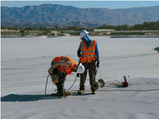
Comanco technicians performing extrusion welding
