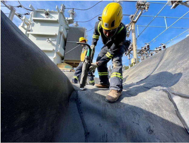
Hallaton Environmental technician extrusion welding HDPE
