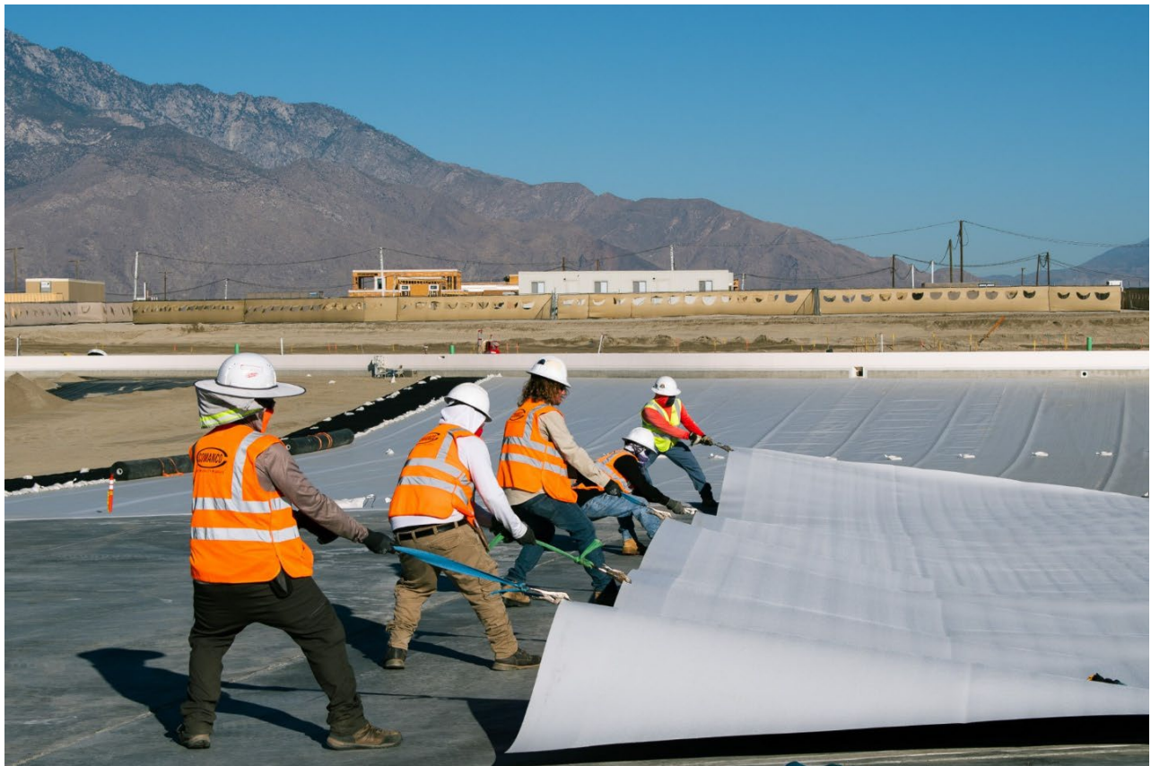
Comanco crew deploying geomembrane sheet for a mining project in USA
