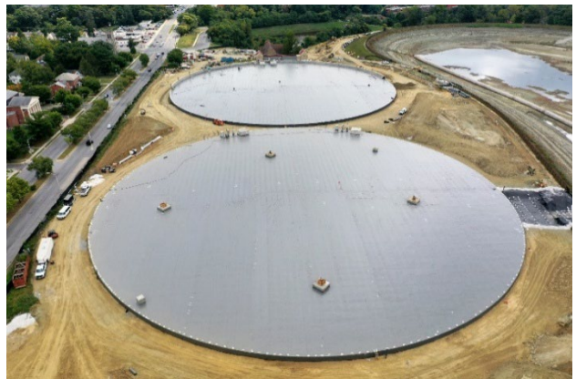
Completed PVC lined tank tops with footings for sports field
